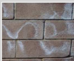
Crystallized efflorescence
